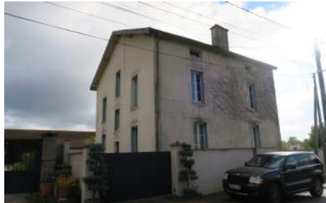
V. BR : Façade, 12 route de Moncel
